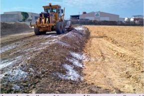
A grader distributes 24 tonnes of lime to neutralise acid sulphate deposits found on the Gladstone building site.
