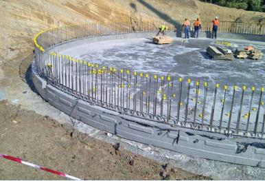
Construction is underway for a one mega-litre underground reinforced concrete reservoir at Lilydale.
